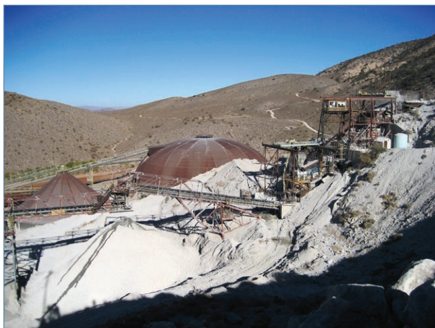
Figure 3. First and second stage crushing circuit with preblending dome in the background.
